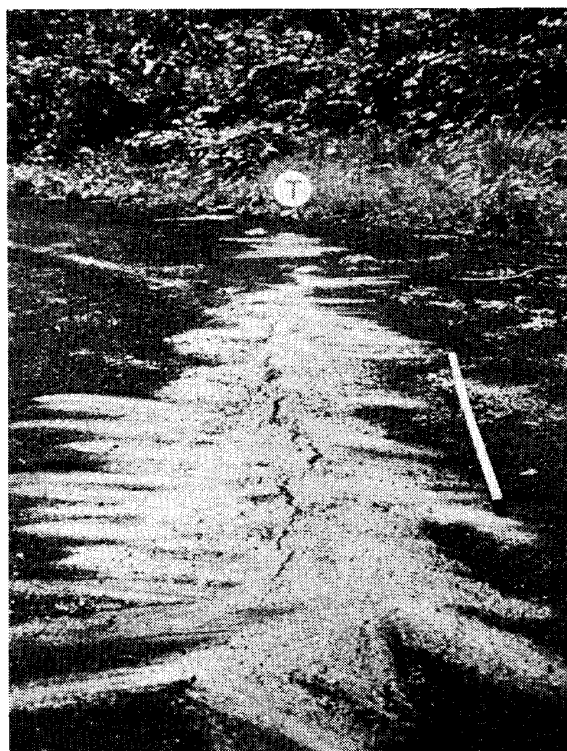
Fig. 19. Crack observed at point X in Fig. 17; 2 cm wide and 2 m long. Photo was taken from the summit side. "T" represents a measuring point of ground temperature.
